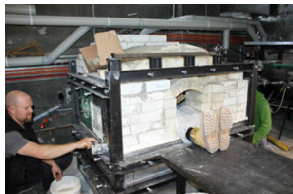
working on the Glassworks tank furnace rebuild
